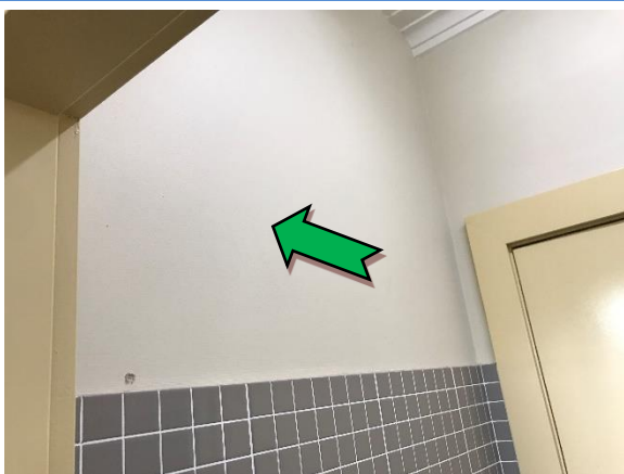
Photo 5. Interior, male and female toilets, wall panels – non asbestos-containing fibre cement sheeting
