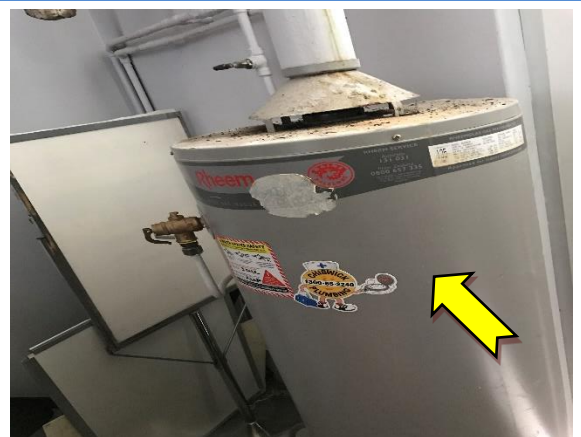
Photo 6. Interior, male change room, hot water heater – suspected SMF internal insulation.
